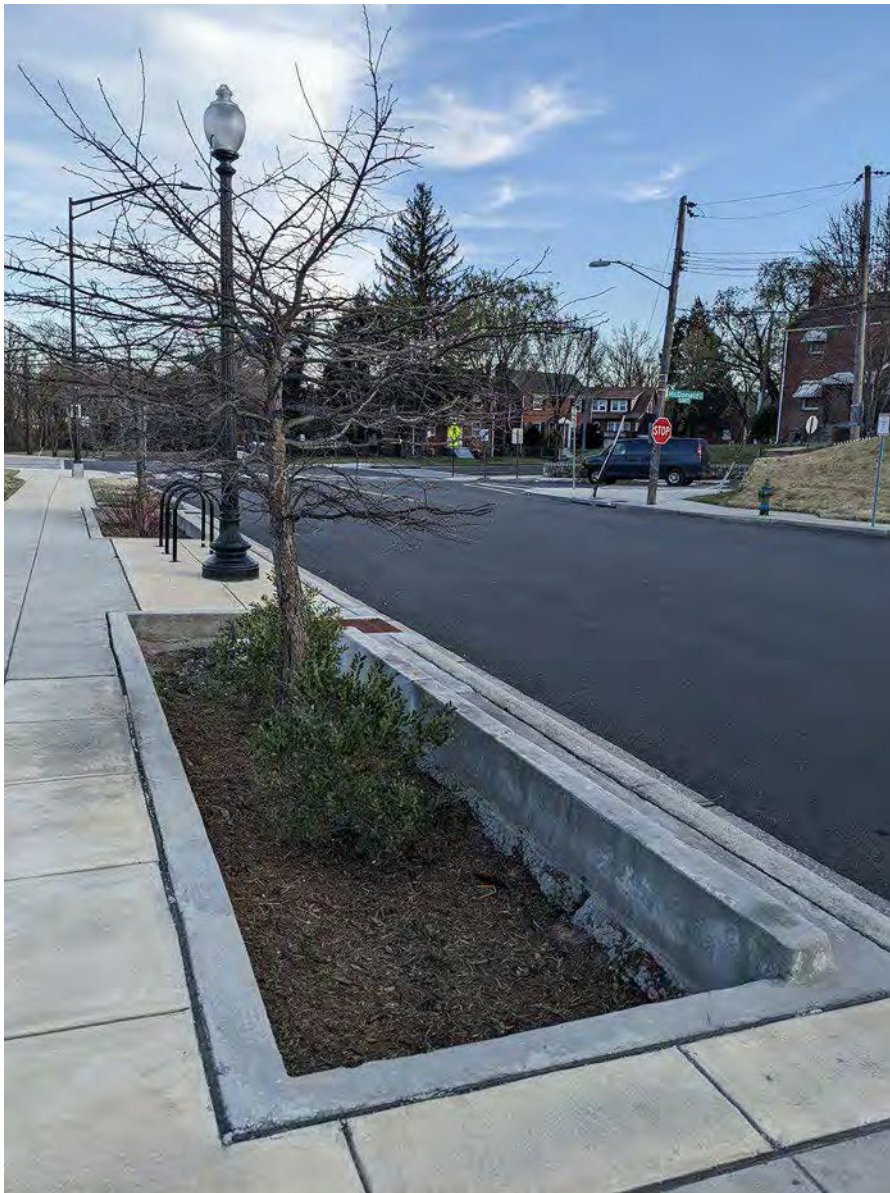
A street-side bioretention planter in Washington, DC.
