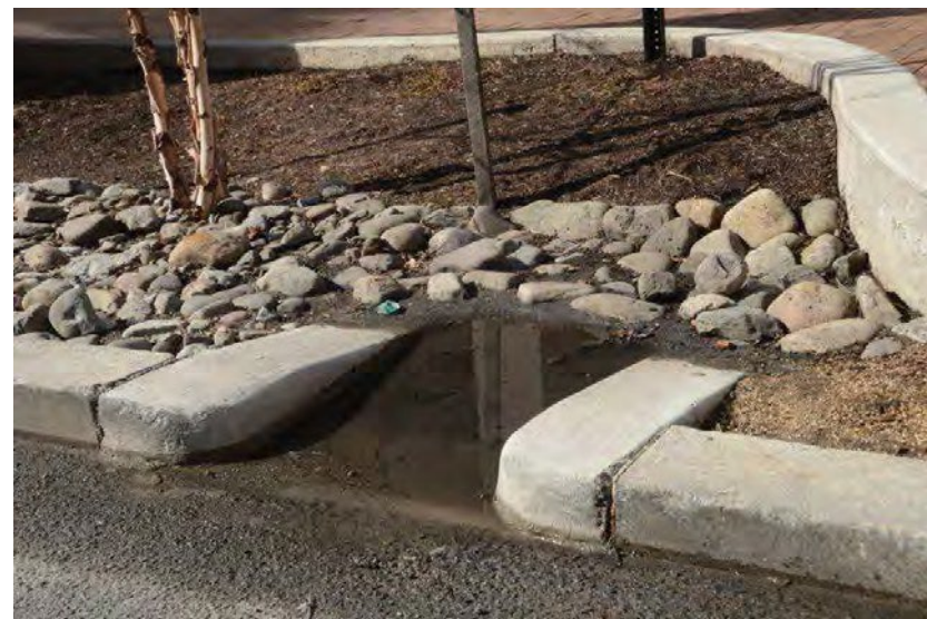
Incorrectly installed inlet.
