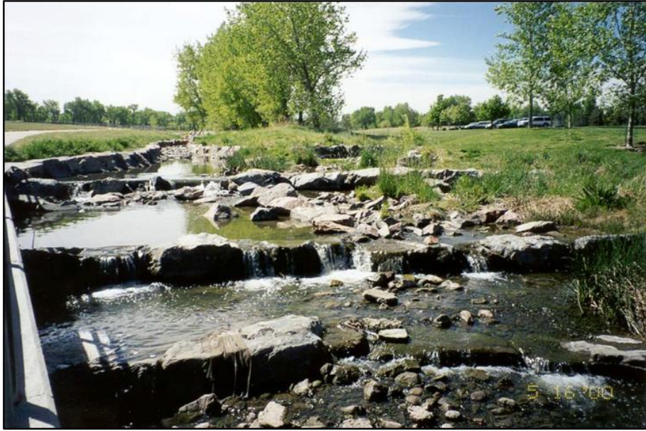
Photograph HS-3 —Stepped grouted sloping boulder drop structures such as in Denver’s Bible Park can be safe, aesthetic, and provide improved aquatic habitat besides performing their primary hydraulic function of energy dissipation.
