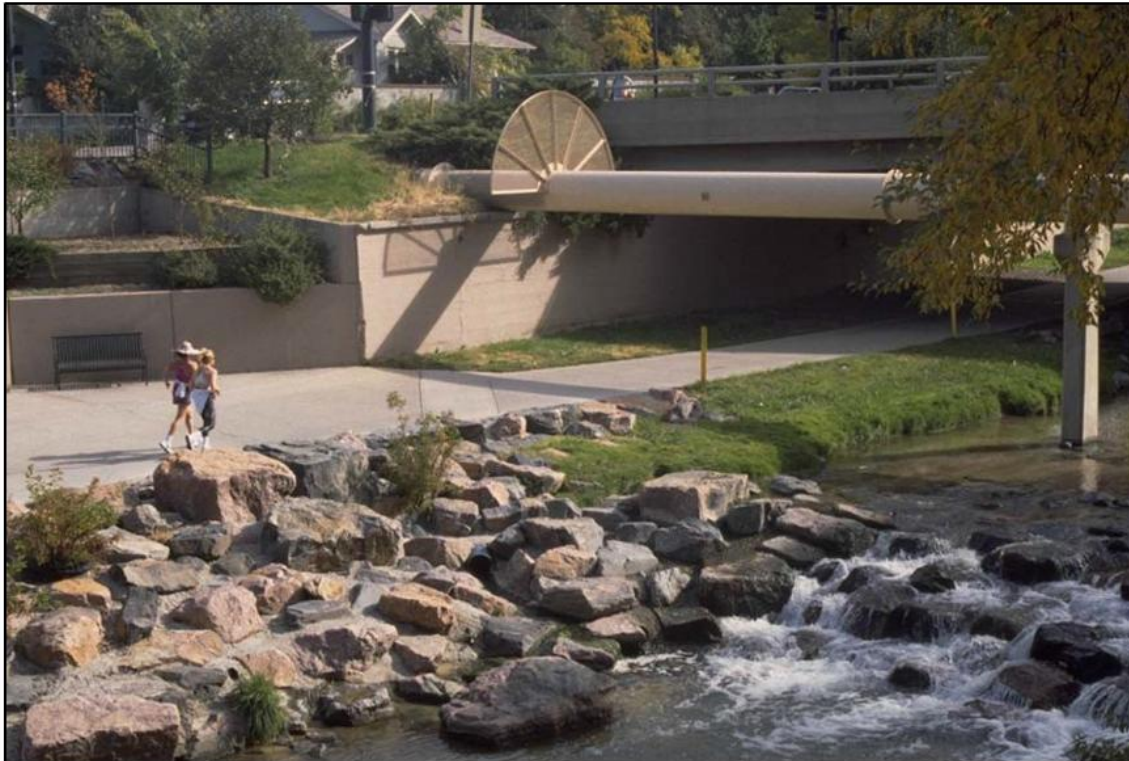
Photograph HS-14. A stable channel at bridges is important and includes caring for the stream downstream of the bridge as shown here on Cherry Creek.
