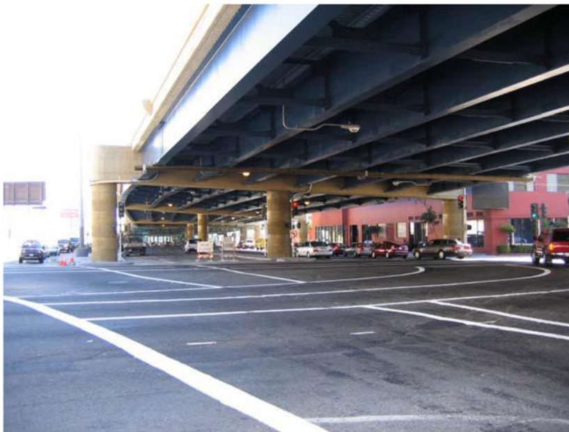
Figure 1.1-1: Central Viaduct in San Francisco
