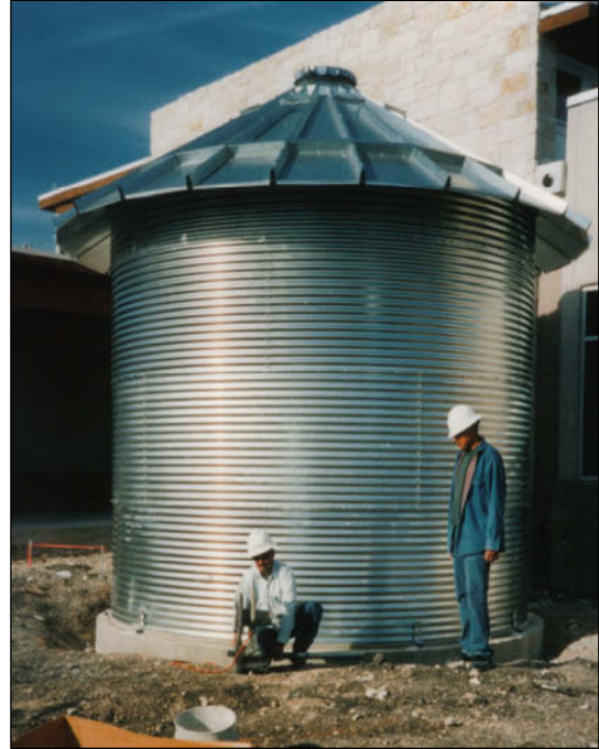
Four lined, galvanized steel tanks will capture water for irrigation of native and adapted plants.
