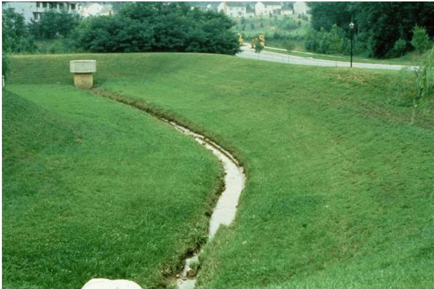
Figure 1-1: Typical Dry Basin
