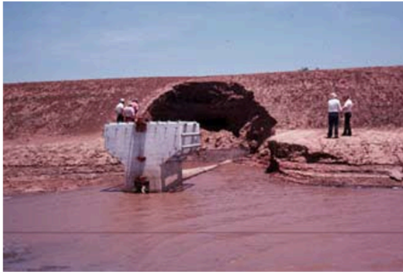
Figure 45–1: Failed embankments
