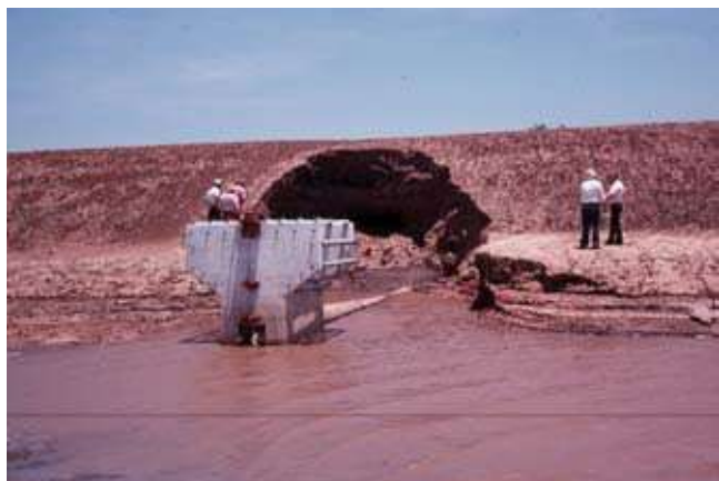
Figure 45-1 Failed embankments
