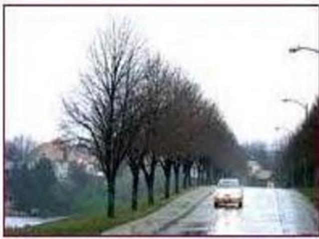
Figure 2. Example dam with problematic trees in Nebraska.
