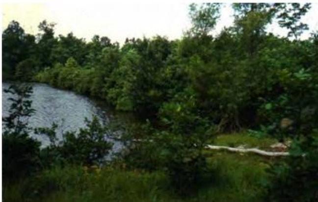
Figure 3. Example dam with inspection- hindering trees in Tennessee.
