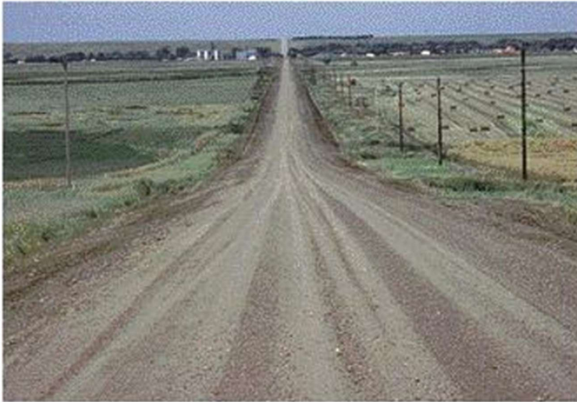
Example of a gravel road with good shape of cross section. Notice crown in driving surface and proper shape of shoulder and ditch.
