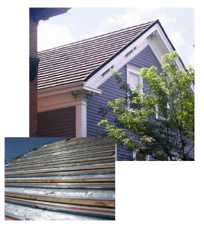
The battens not only provided a casing for the solar product, they also solved another problem: the stability of the roof frame and the uneven deck. The battens leveled the roof and provided structural integrity and shear strength.
