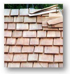
Because of this fire-proofing and other preservatives added to the wood in the manufacturing process, the water from a wood roof is not potable because the preservatives can leach heavy metals, in particular arsenic.
