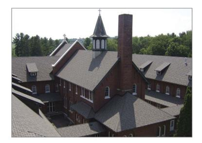
Since the fiber cement tiles were heavy (500 lbs. per square), any additional weight added to the roof structure would need to be minimal.
