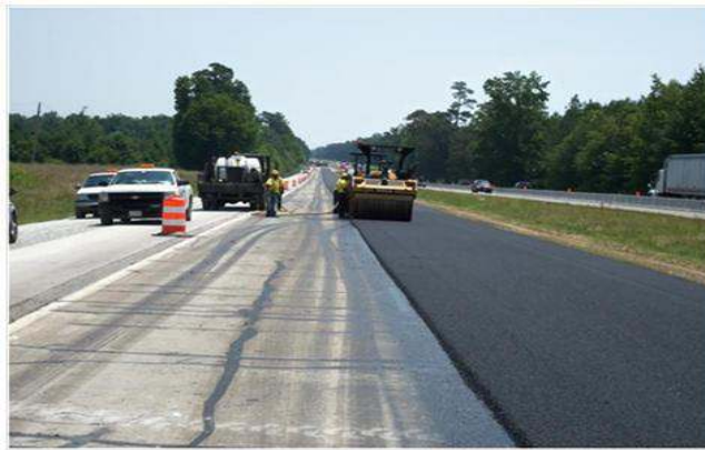
Figure 20. Unbonded overlay on U.S. Route 58 in Virginia. Placement of AC porous friction course.
