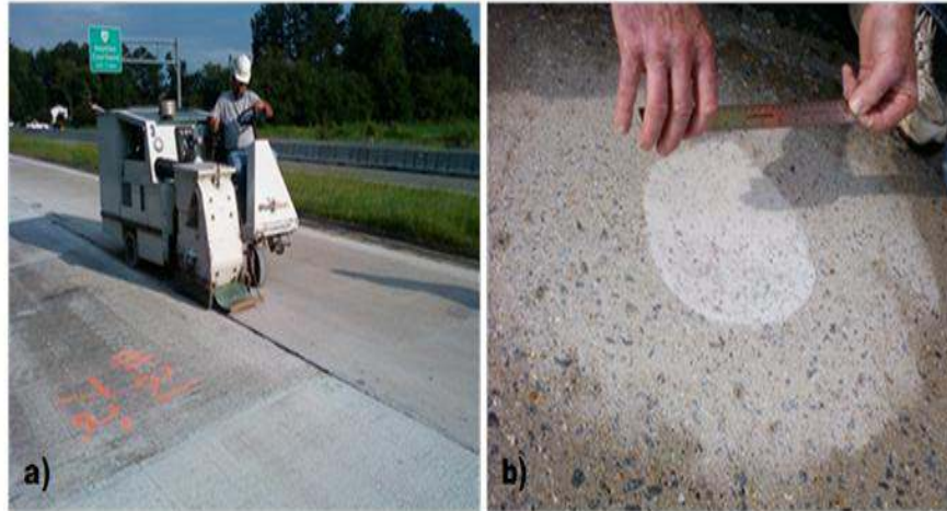
Figure 18. a) Surface preparation for bonded overlay on U.S. Route 58 in Virginia; b) Closeup view of surface after preparation.
