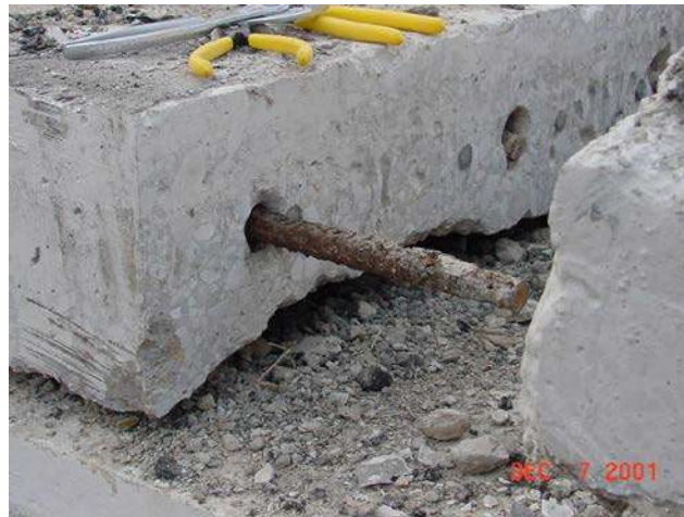
Figure 10. Lack of bond between inserted rebar and concrete. (20)
