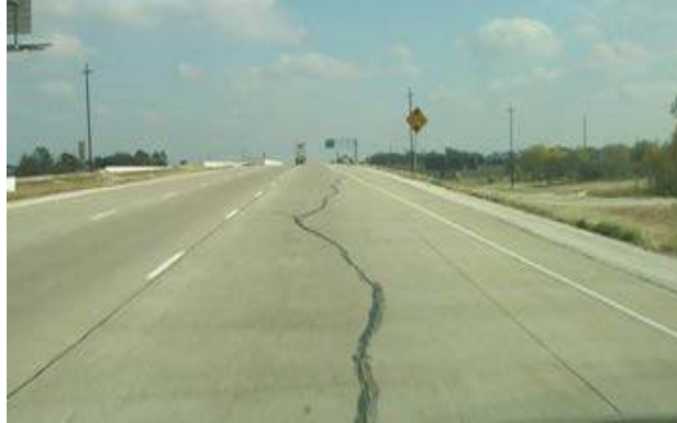
Figure 1. Longitudinal crack in CRCP.
