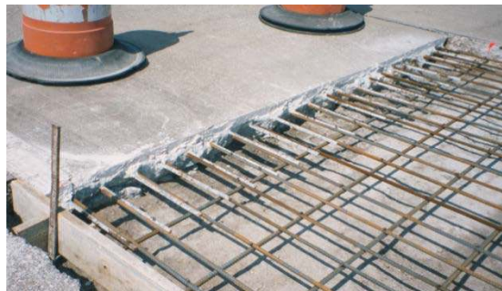
Figure 9. Maintaining reinforcing steel continuity in CRCP. (1)
