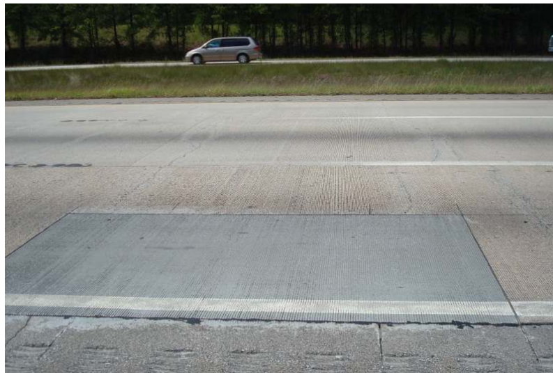
Figure 13. Half-lane-width FDR on I-77 in South Carolina.
