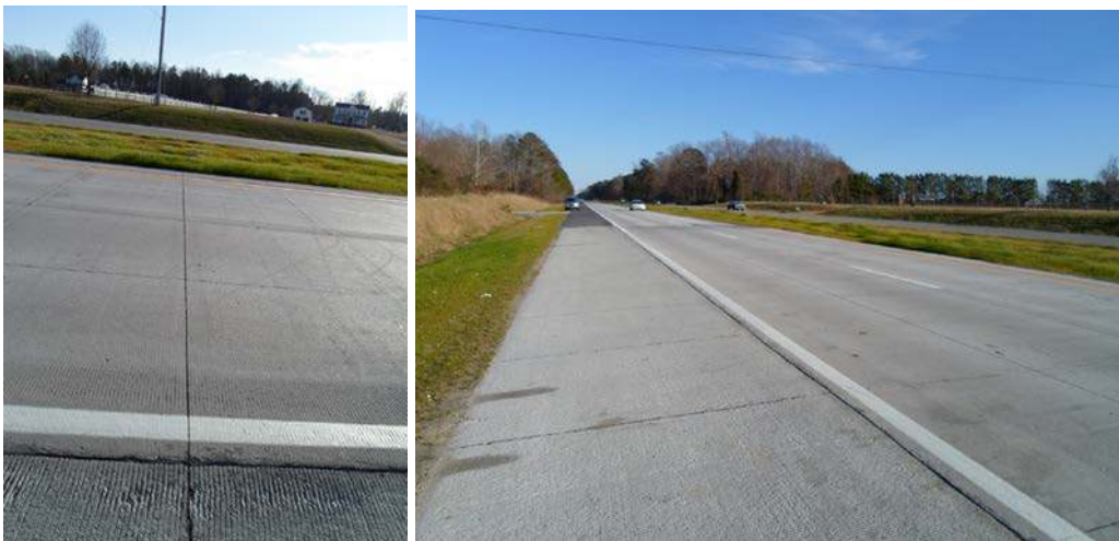
Figure 21. Unbonded overlay on U.S. Route 58 in Virginia, as constructed, with 6 ft by 6 ft joint layout.
