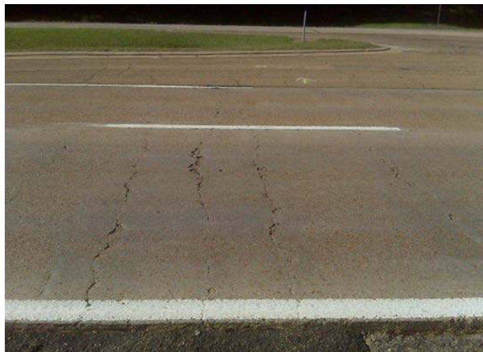
Figure 3. Spalling at CRCP transverse cracks.
