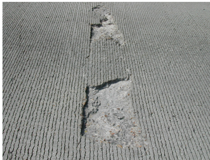
Figure 15. Shallow spall. (19)
