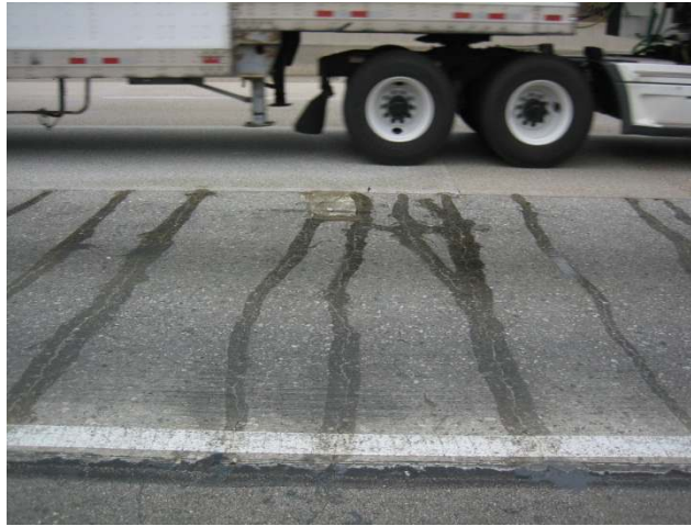
Figure 16. Epoxy sealing of CRCP cracks.
