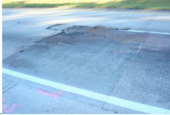
Figure 14. Failure of FDR.
