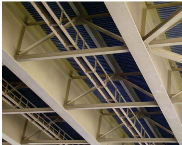
Figure 2 Photo of a typical girder substringer system showing a stringer sitting on top of cross frames
