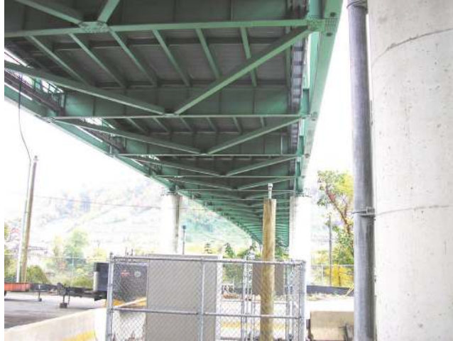
Figure 6 Photo showing a typical stacked floor system
