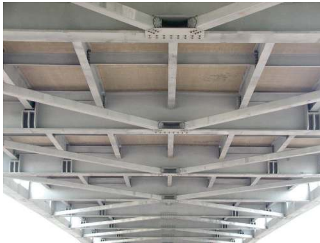
Figure 7 Photo of a typical framed floor system
