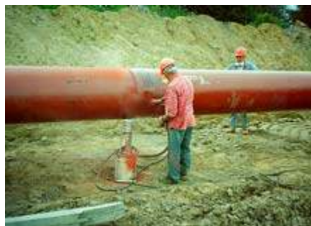
FIGURE 3.3-12 Applying Coating to Pipeline
