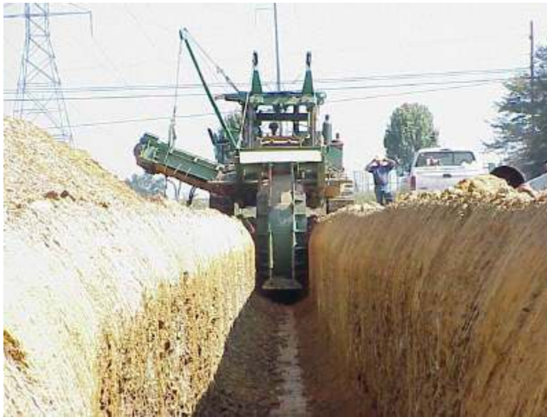
FIGURE 3.3-9 Pipeline Ditching (Source: Photo courtesy of U.S. Pipeline, Inc. Reproduced with permission.)
