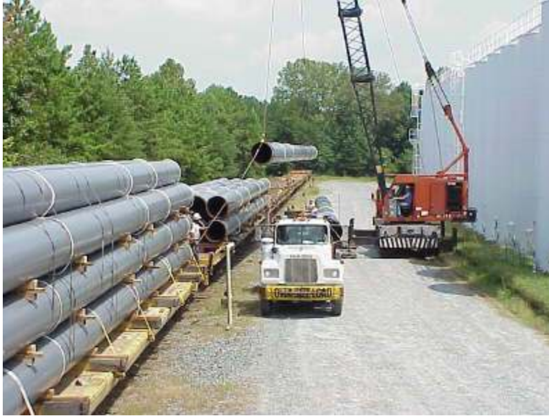
FIGURE 3.3-4 Pipe Segments Arriving at Rail Off-loading Area (Source: Photo courtesy of U.S. Pipeline, Inc. Reproduced with permission.)
