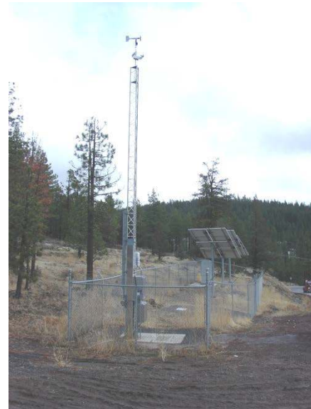
Figure CA-2. Road weather information system at Fredonyer East ICWSs.
