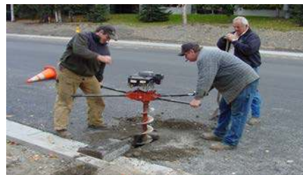
Figure AK-2. Boring hole for temperature probe.
