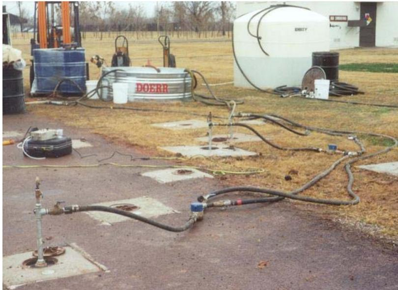
**Figure 5.6 Typical Injection System Using a Field Prepared Emulsion, Altus AFB, Oklahoma**
