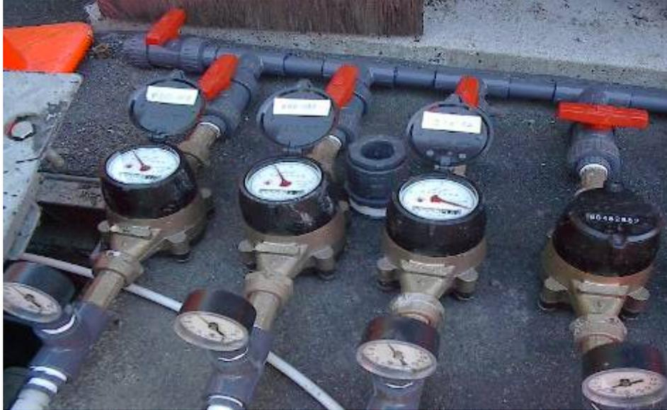
**Figure 5.10 Injection System Manifold Showing Separate Control Valve and Flow Totalizer for Each Injection Well** (Photo courtesy of EOS Remediation, Inc.)
