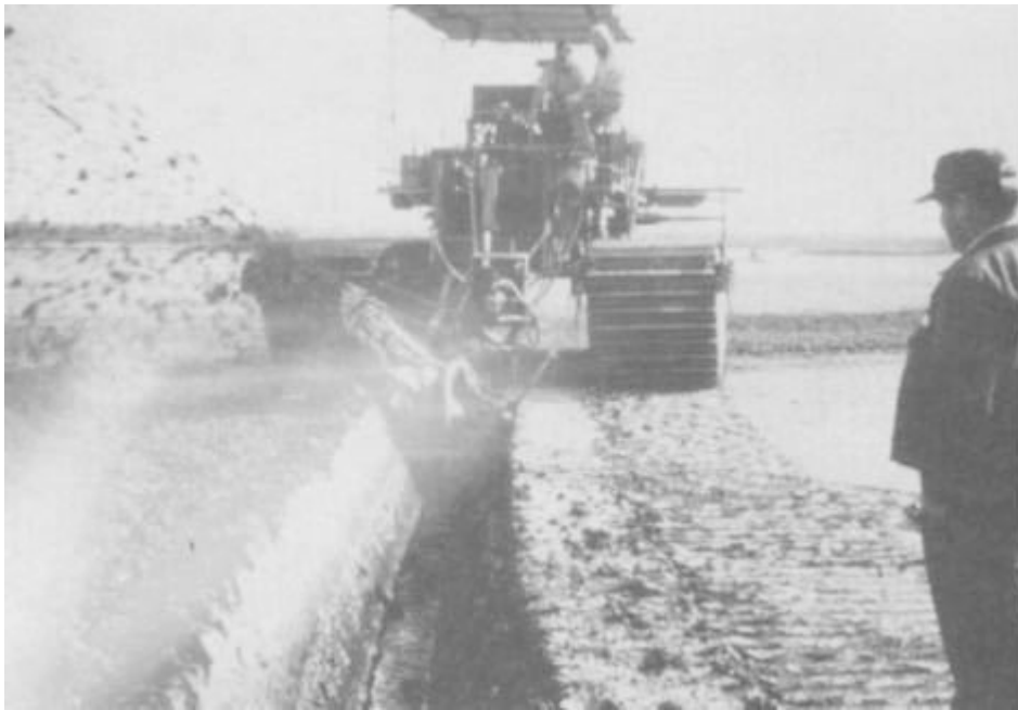
Figure 5-19. View of rotary trenching device in operation
