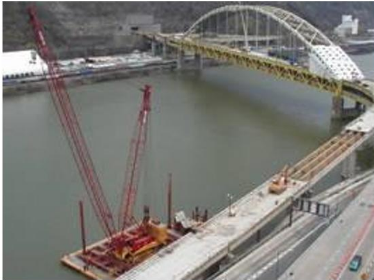
Figure 4: Photograph of a lattice ringer crane
