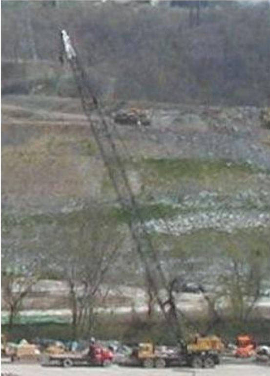
Figure 2: Photograph of a mobile lattice boom crane
