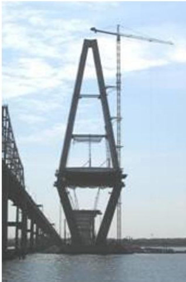
Figure 5: Photograph of a tower crane
