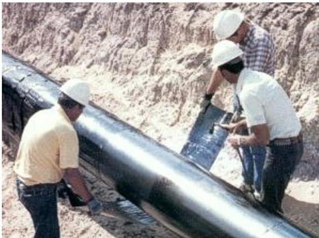
Figure 2.1-1: Coating Newly Installed Pipe for Corrosion Control (Source: Photo courtesy of Corrosion Control Products Co. Reproduced with permission.)
