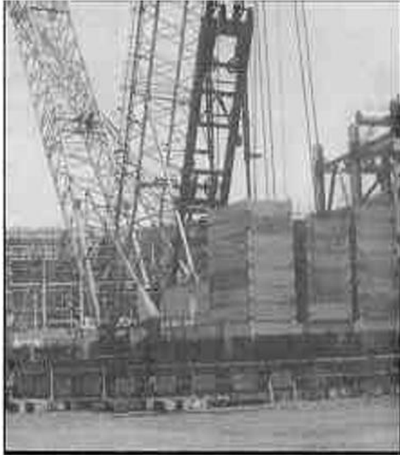
Figure: Modern Ringer Crane 500 Ton Capacity
