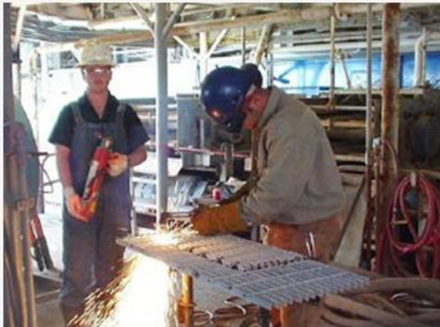
Figure 1. Hot work - welding
