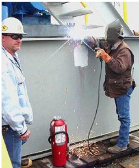
Figure 2. Welding with fire control
