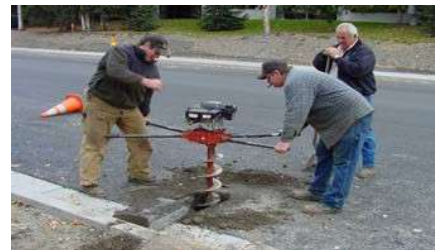
Figure AK-2. Boring hole for temperature probe.
