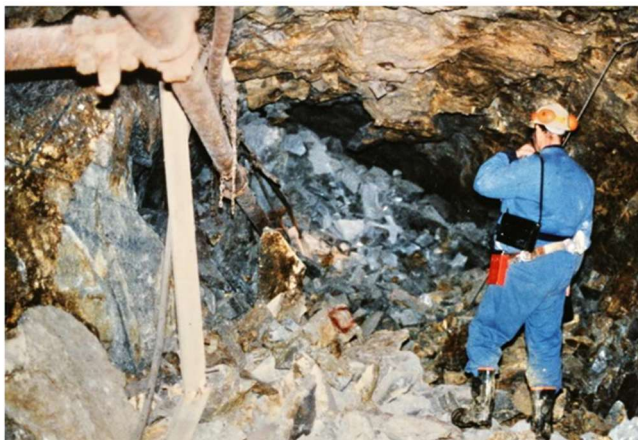
Figure 3: The results of a rockburst in an underground mine in brittle rock subjected to very high stresses.
