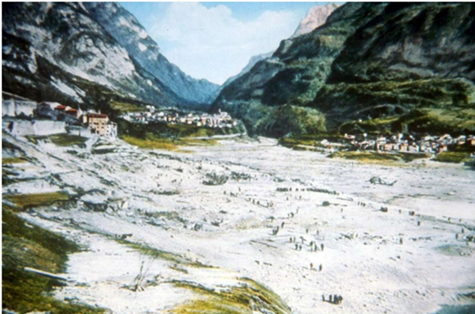
Figure 2d: The remains of the town of Longarone after the flood caused by the overtopping of the Vajont dam as a result of the Mount Toc failure. More than 2000 persons were killed in this flood.
