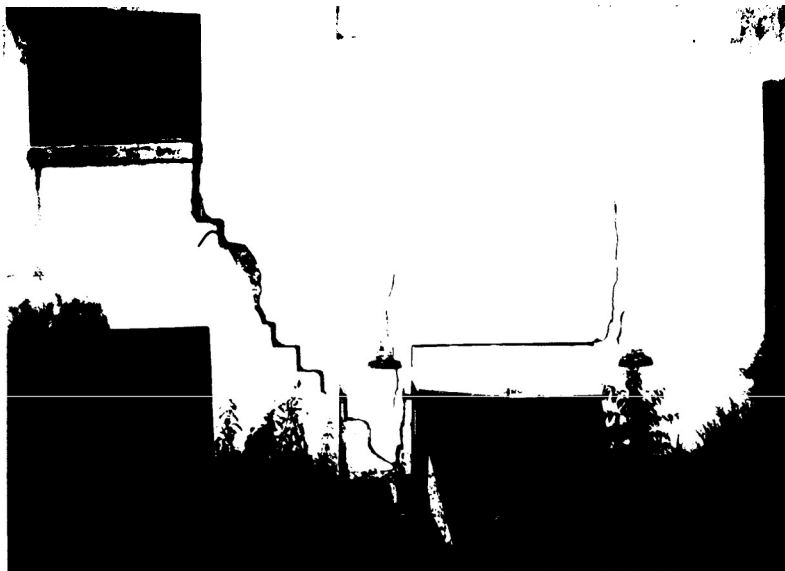
Figure 1-1. Examples of cracks in an exterior wall.
