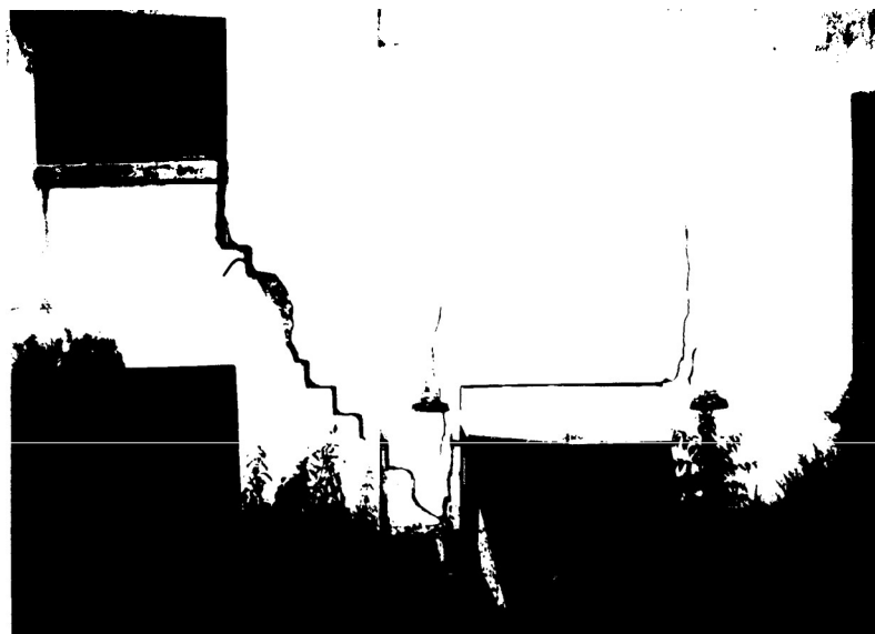
Figure 1-1. Examples of cracks in an exterior wall.
