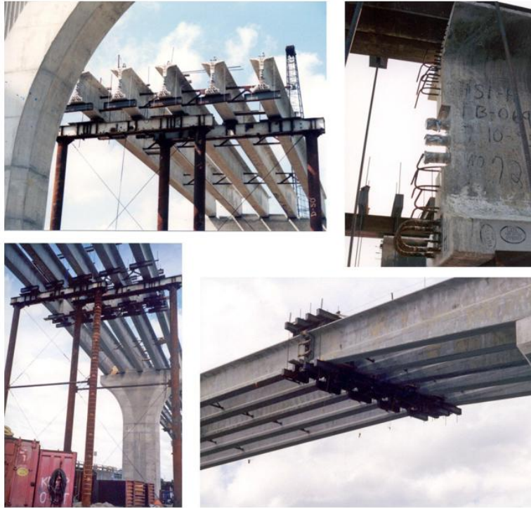
Figure 1.7. Spliced Haunched I-Girder of Main Span Unit
