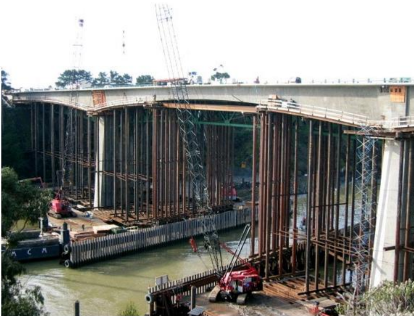
Figure 1.6. Cast-In-Place Post-Tensioned Construction in California
