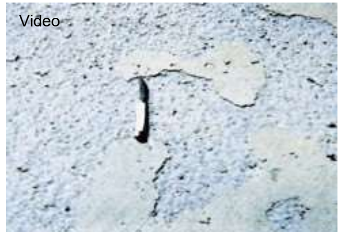
Fig. 6-3. Scaled concrete surface resulting from lack of air entrainment, use of deicers, and poor finishing and curing practices. (52742)
