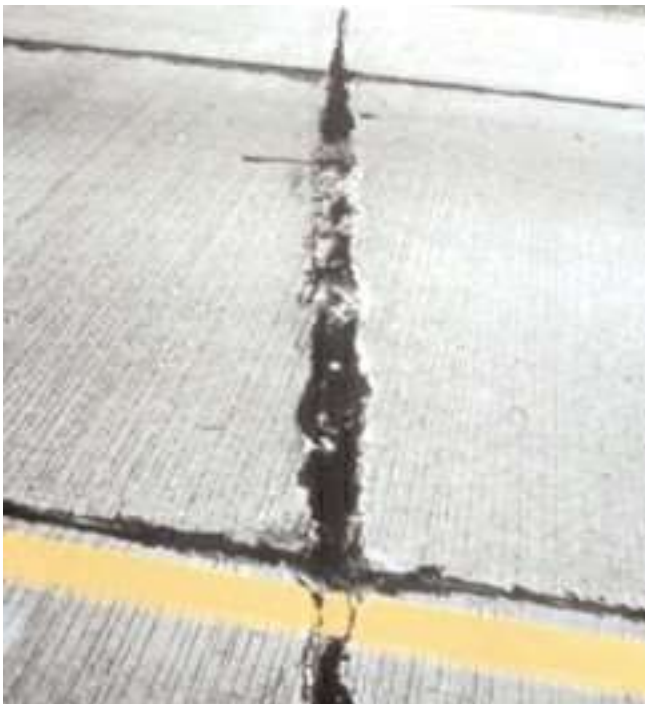
Fig. 6-3. Scaled concrete surface resulting from lack of air entrainment, use of deicers, and poor finishing and curing practices. (52742)
