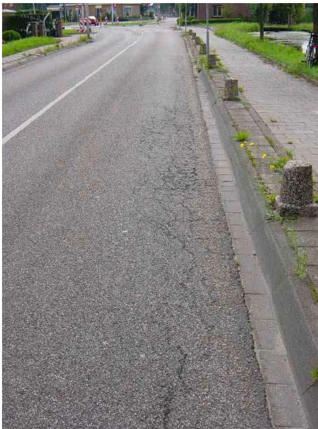
Figure 2: Longitudinal and alligator cracking in the Wheel path.
